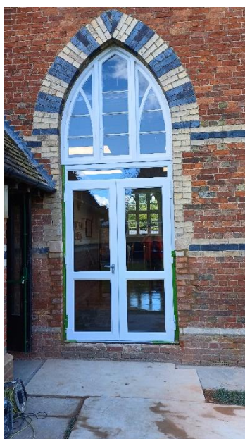
Internal and external views of the new garden door being fitted
