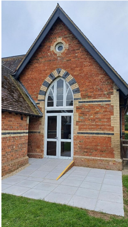
New double door fire exit and wheelchair ramp to rear garden
